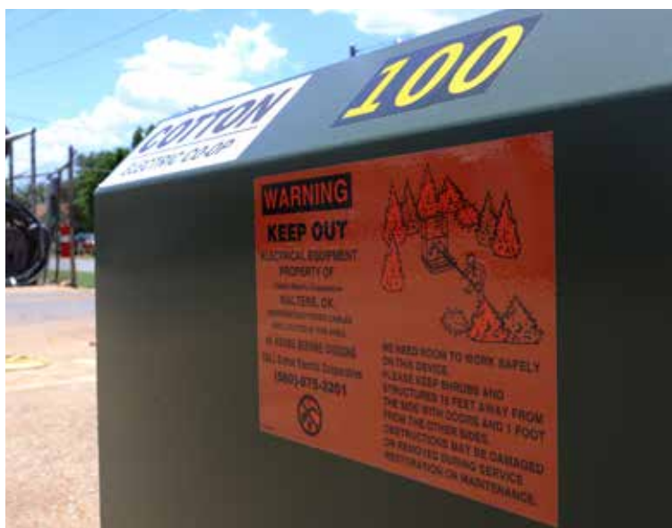
Every pad-mounted transformer provided by Cotton Electric comes with an orange sticker explaining how to stay safe around the equipment. Photo by Carli Eubank.
